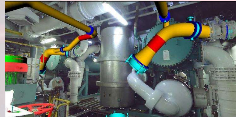
AC Chiller 3D piping interface modeling and 3d model overlap on existing compressor room environment
